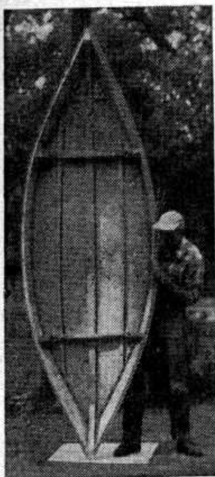
Fig. 4. Hull with bottom complete removed from form.
